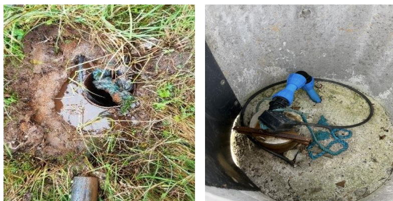
Figure 1: poorly (left) and properly (right) constructed well.
